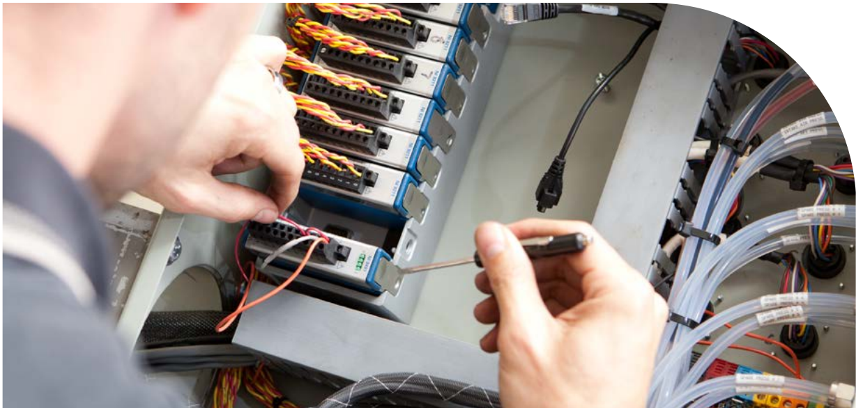
FIG 5 | Standardize on a few module connectors (screw terminals shown in image above) for efficient system assembly and support.
