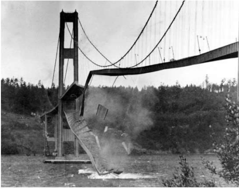
Figure 1. Structures may fail if their natural frequencies match environmental vibration.
